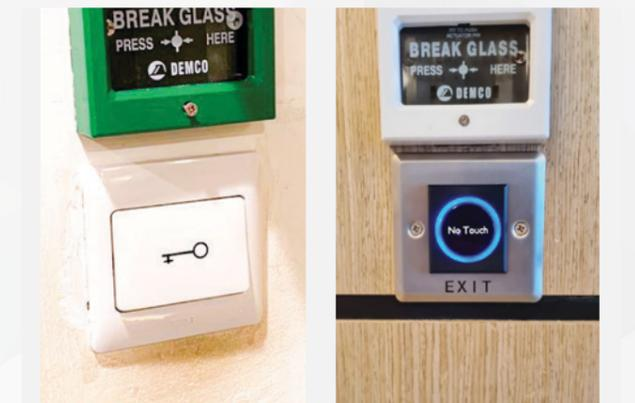
Exit buttons have been replaced with contactless sensors, reducing the risk of transmission.
