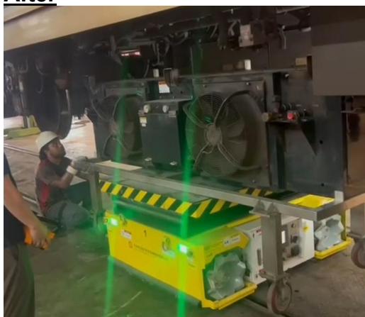
Photo of staff operating the remote-controlled lifting table to install parts underneath the train
