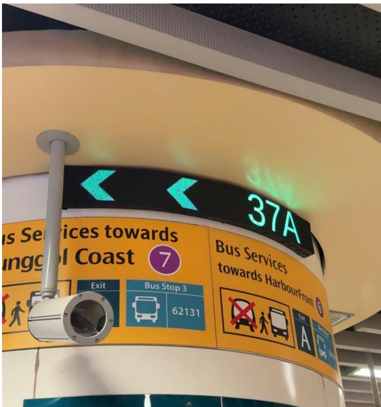
Photos 4, 5, 6: Flashing arrows are activated for commuters in the event that disruptions occur, to guide them to the closest exit or bus bridging points.
