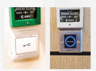
Exit buttons have been replaced with contactless sensors, reducing the risk of transmission.
