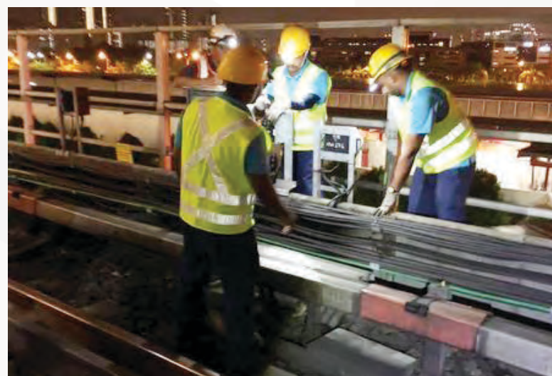
Replacing track circuits on the NSEWL which will automatically detect broken rails.
