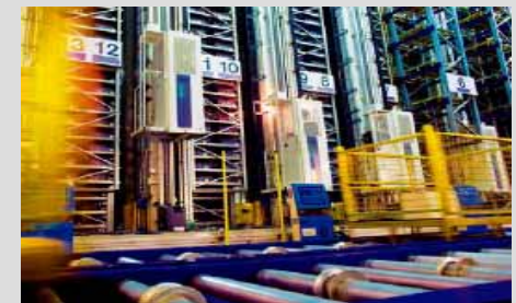
Engineering Consultancy & Services
